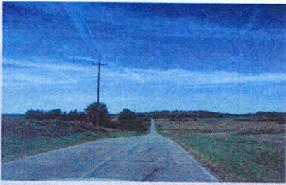
Power lines on one side of road, minimal grade change
