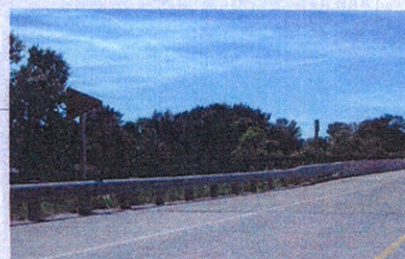
Snowmobile bridge adjacent to Highway 19
