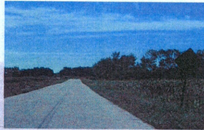
Narrow ROW and no shoulder on Island Road
