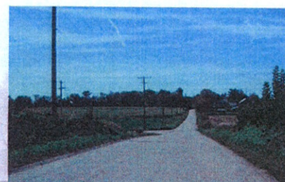
Hubbleton Road: More narrow, less traffic
